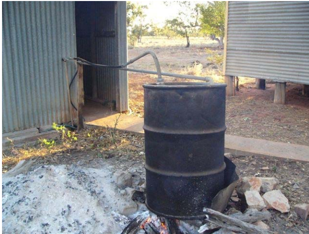
The hot water system for the showers & spa
